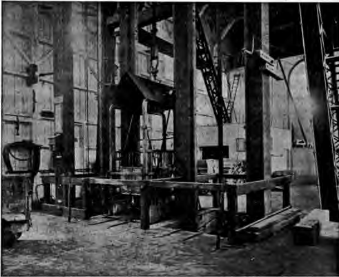
Landing at the top of a mine shaft.
